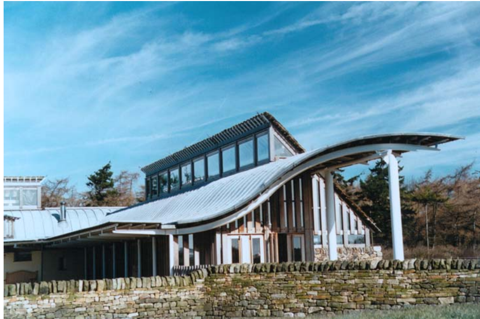
Figure 1.1 Single storey structure with curved roof
