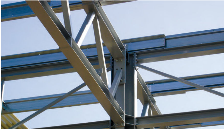
Figure 3.25 Truss-column connection in a rigid framed structure
