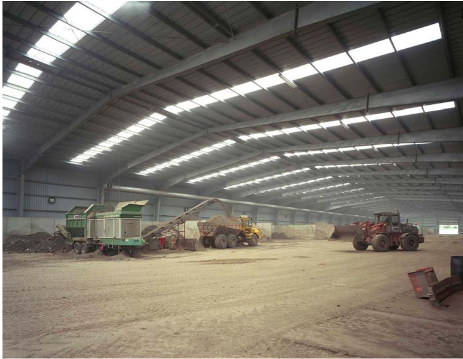
Figure 3.3 Pitched roof portal frame
