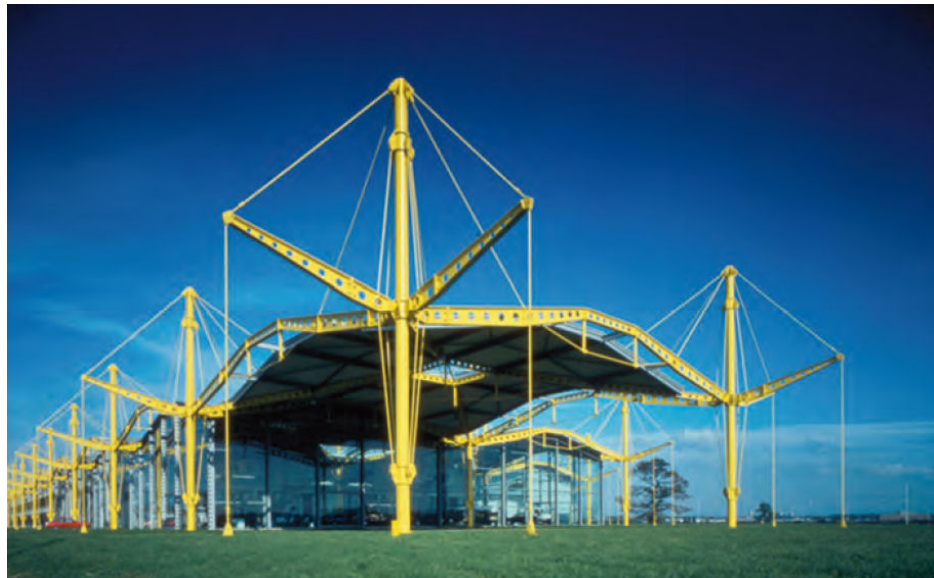
Figure 2.4 Dramatic, expressed steelwork
