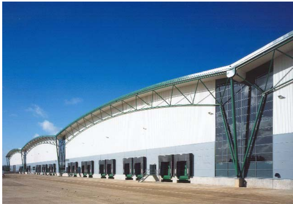
Figure 1.2 Single storey warehouse with exposed steelwork truss
