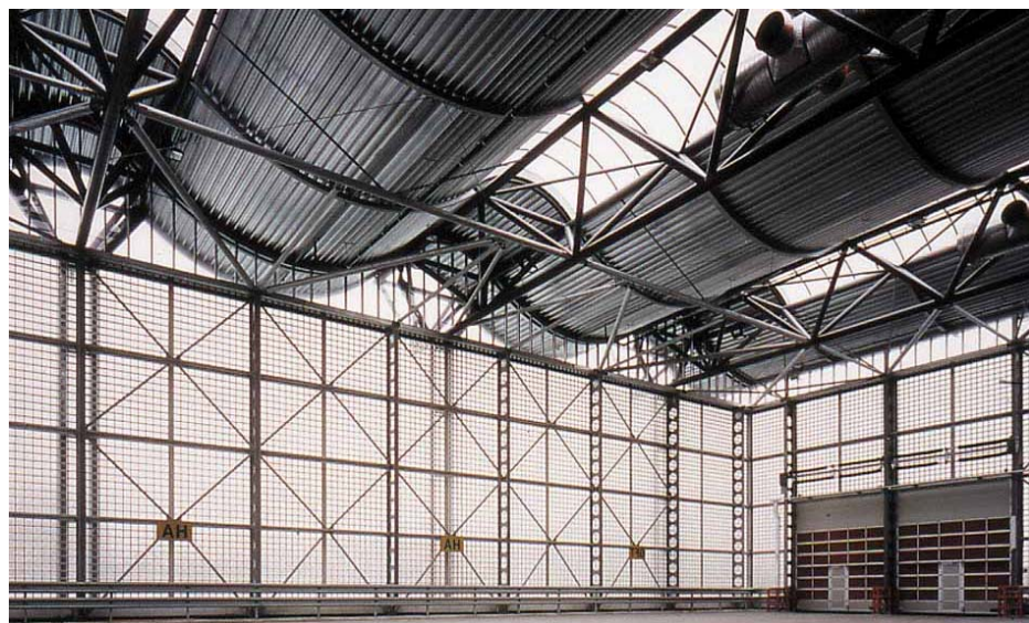
Figure 3.19 Three-dimensional trusses supporting a roof
