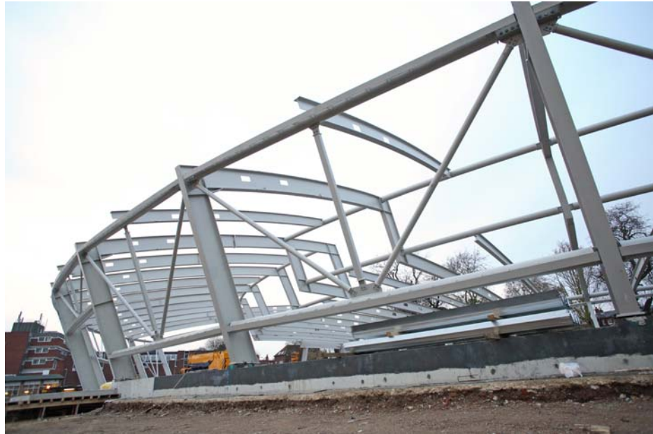
Figure 1.3 Single storey curved and cranked steelwork for an art gallery
