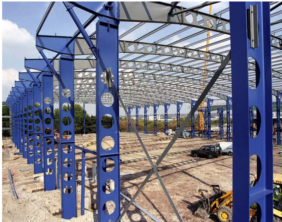
Figure 2.1 The relatively low self weight of steel structures reduces material delivery to site
