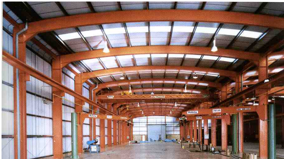
Figure 3.4 Curved roof portal frame
