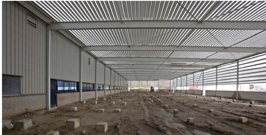
Figure 3.12 Pinned frame beam and column structure
