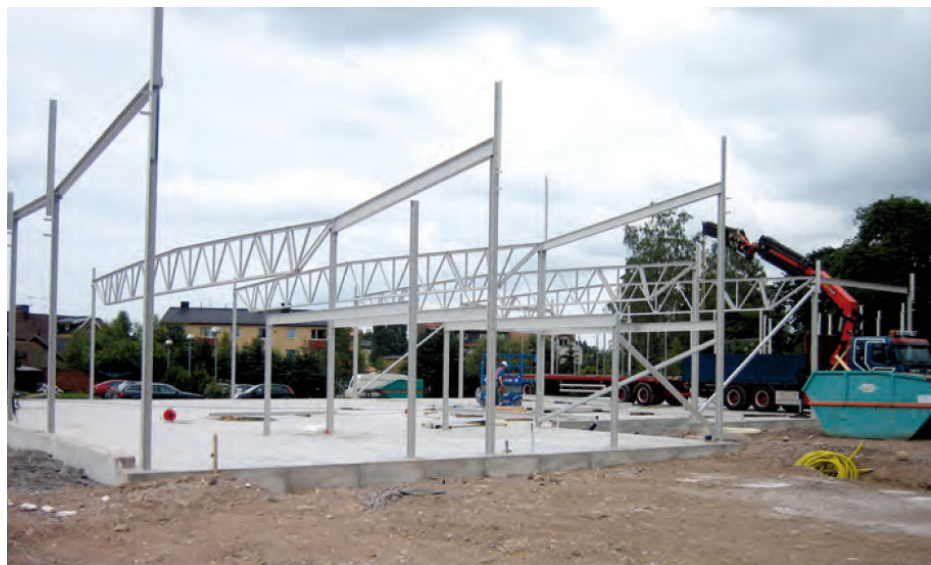
Figure 3.17 Flat truss in pinned frame building
