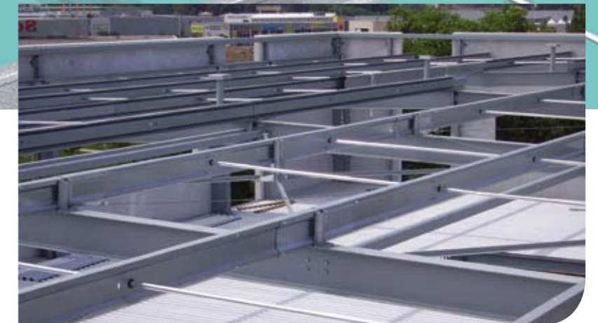
Multibeam on a steel structure
