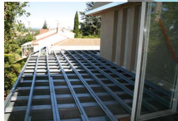
Joists between bars and over bars
