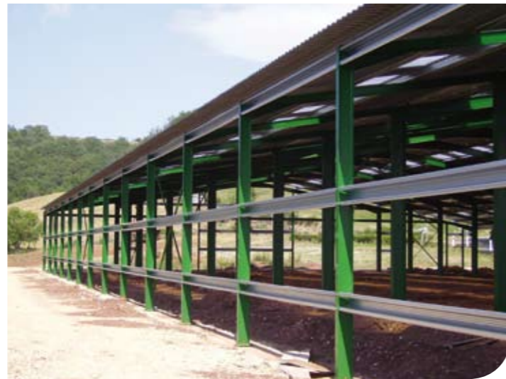
Principle for fitting rails onto inside of stanchions
