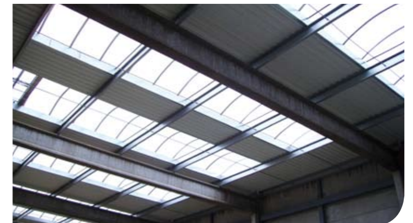
Multibeam on a concrete structure
