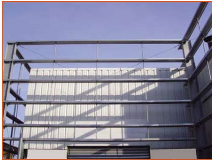
Rail system between and in front of stanchions
