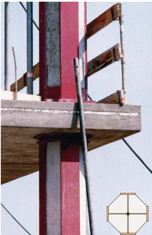
Figure 22: cross-shaped column filled with concrete
