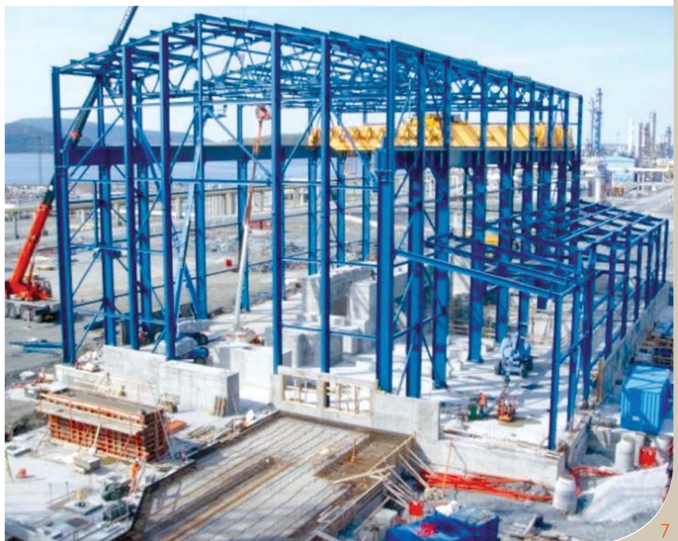
Figure 6: SIEMENS Combined Cycle Power Plant - steel structure of the power houses
