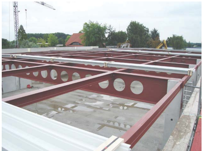
Figure 25: ease of installation of ACB beams
