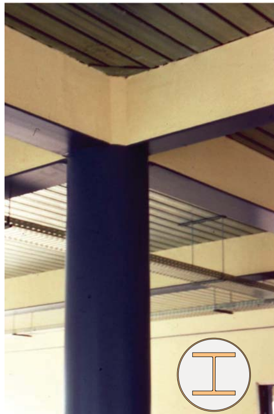
Figure 23: concrete-filled pipe with an embedded rolled section
