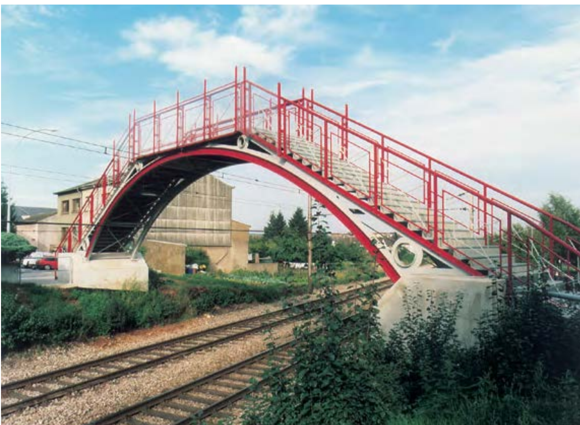
Footbridge near Schiffflange, Luxembourg – Principle beams with an extreme curvature.
