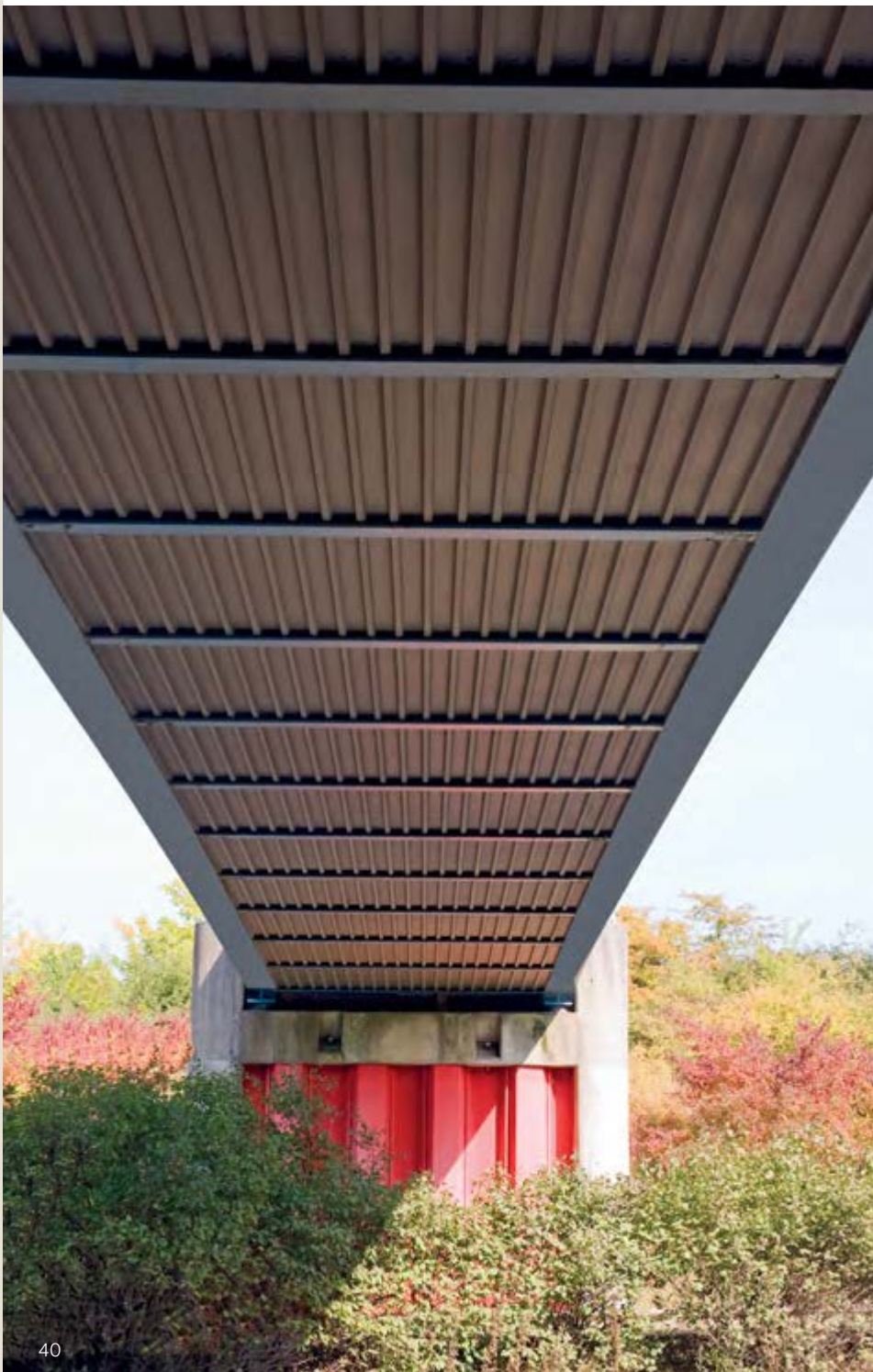
Bottom view on the footbridge at Soleuvre, Luxembourg – Sheet piles are used for the abutments.
