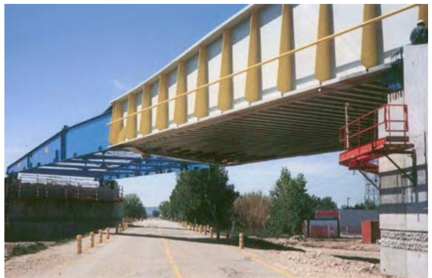
A half-through girder deck during launching. It carries the new Mediterranean High Speed Railway Line which was opened to traffic in 2002. The exposed flanges of the transverse filler beams can be seen at the bottom side. The blue coloured part is the launching nose.
