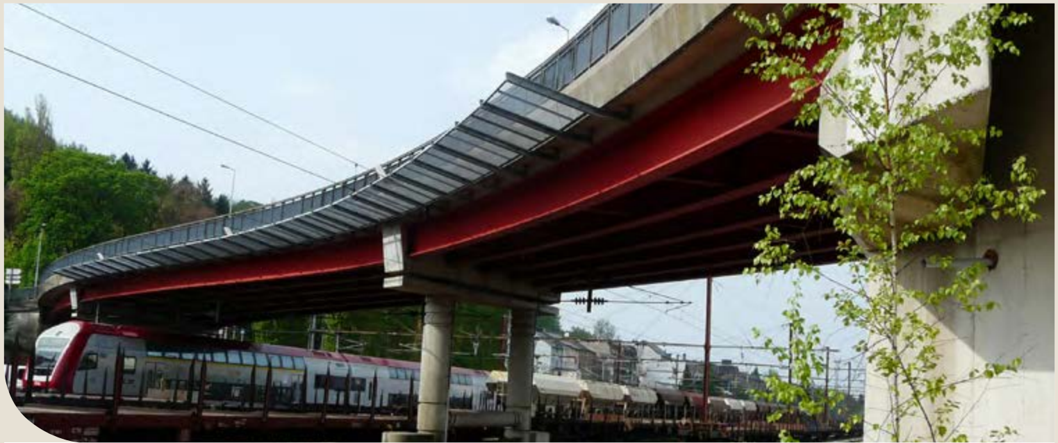
Roadbridge in Differdange, Luxembourg – Bridge with a strong bending over the weak axis (see erection of two main girders on page 9).
