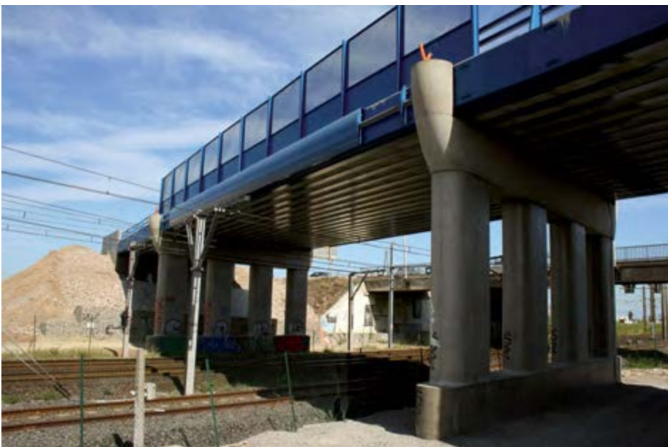
Railway bridge at Sète-Frontignan, France
