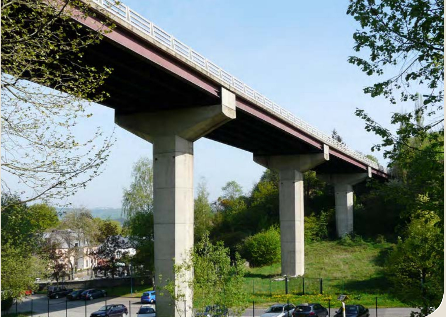
Multiple span viaduct at Ditgesbaach, Luxembourg
