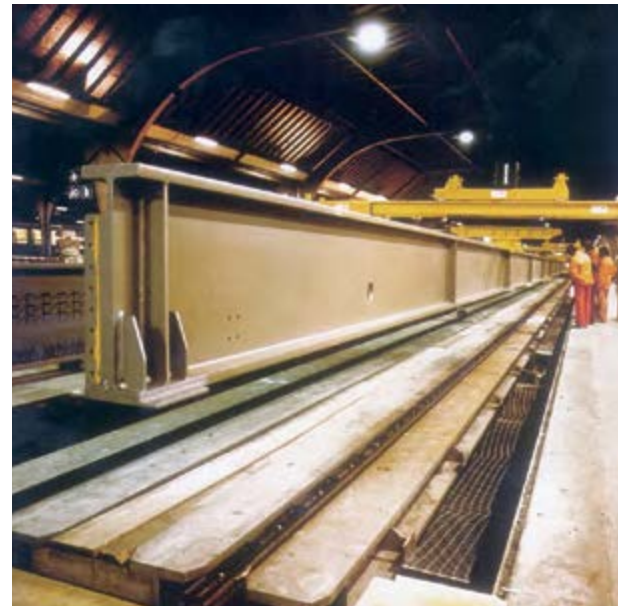
Renovation of the platform in the main station in Zürich – The new 5-span decks for ballasted track are of half through girder type with rolled beams and a reinforced concrete slab supported on lower flanges. Available time and space dictated the erection procedure. The 69 m long beams were lifted into position with portal cranes.
