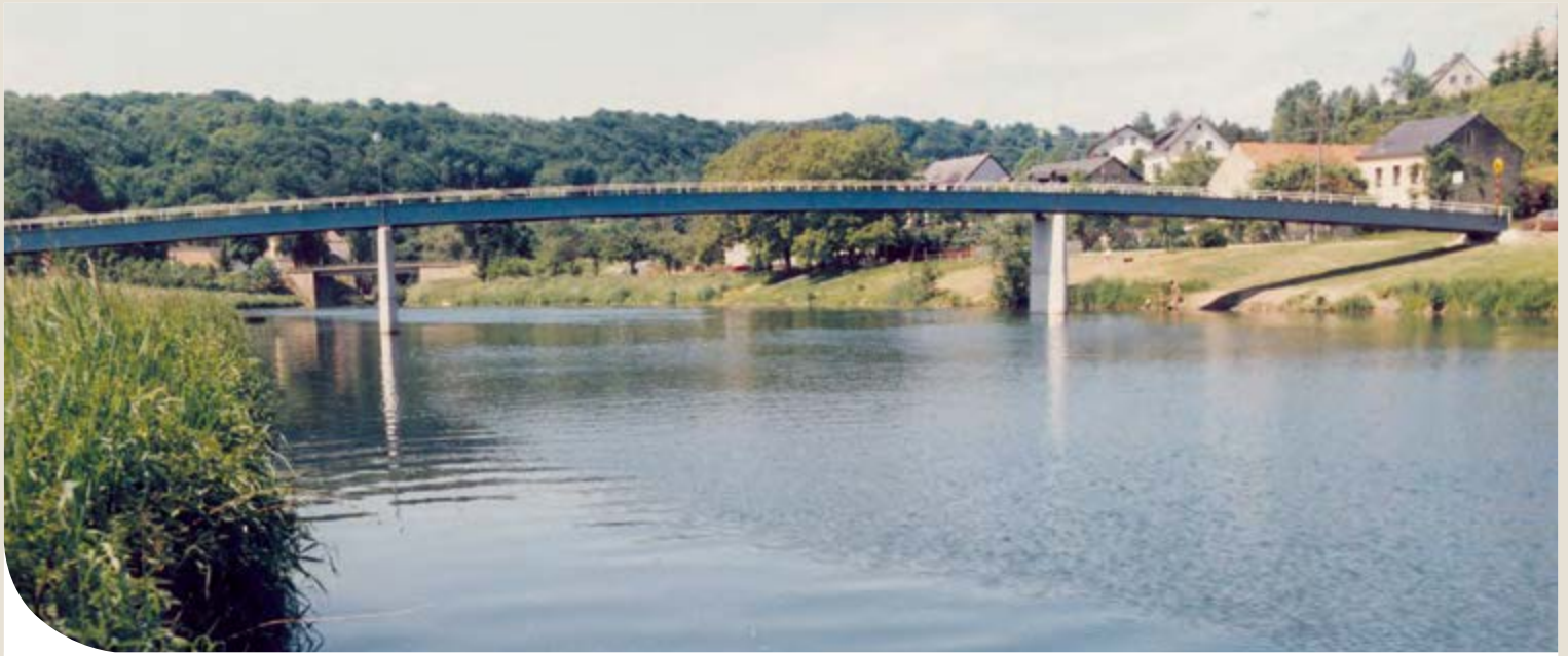
Footbridge over the Sûre at Steinheim, Luxembourg
