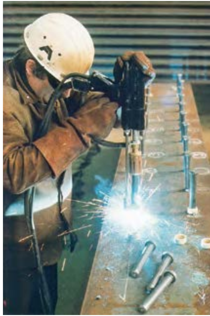
Finishing workshop - Welding of shear stud connectors.
