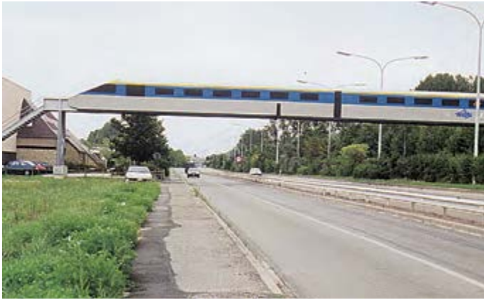
Footbridge for the visitors of a leisure park in Wavre, Belgium - Through type bridge with thematic enclosure.
