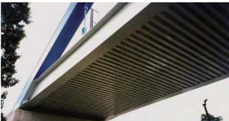
This example shows a bow-string bridge for the Mediterranean high speed railway line over the French highway A7 near Avignon (F). A filler beam deck has been used to span transversally to the bridge axis.
