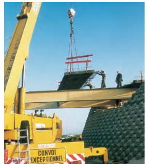
Prefabricated slab - erection of a precast concrete element
