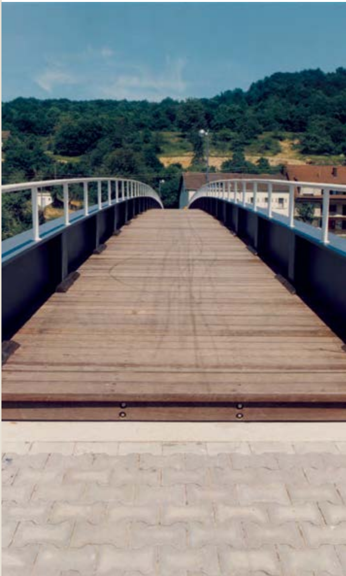
View on the wooden walkway of the half-through bridge with rolled sections in Steinheim, Luxembourg
