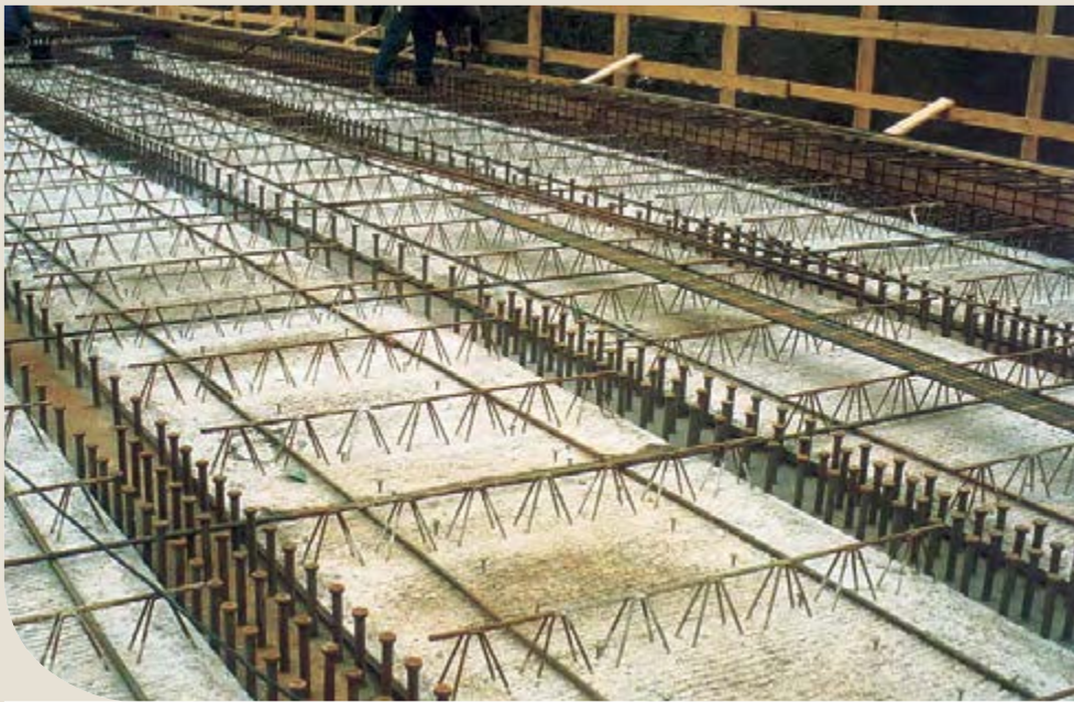
Precast reinforced concrete panels used for permanent formwork.
