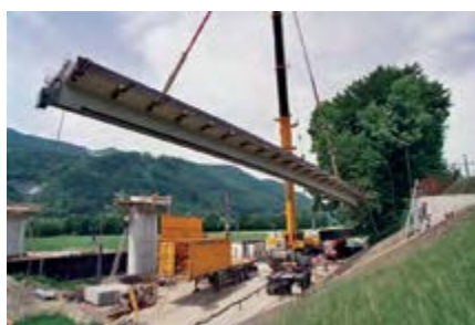
Lifting-in of a PreCoBeam for the bridge at Vigaun, Austria.
