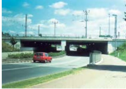
Multiple track railway bridge in Nienburg, Germany - The longitudinal profile of the road and the tracks greatly restrict the available construction depth.
