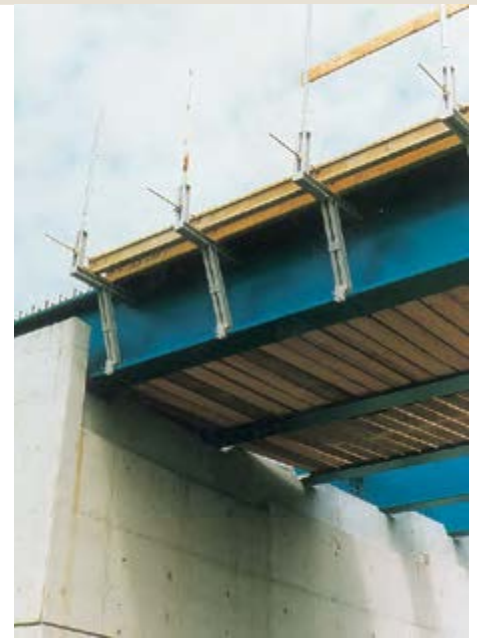
Ex. of formwork support for cantilever part of slab.
