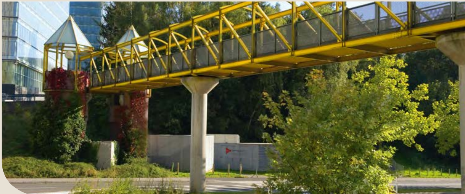
Access footbridge to the building of the Court of Justice of the European Union, Luxembourg – Architectural design based on lattice girders.
