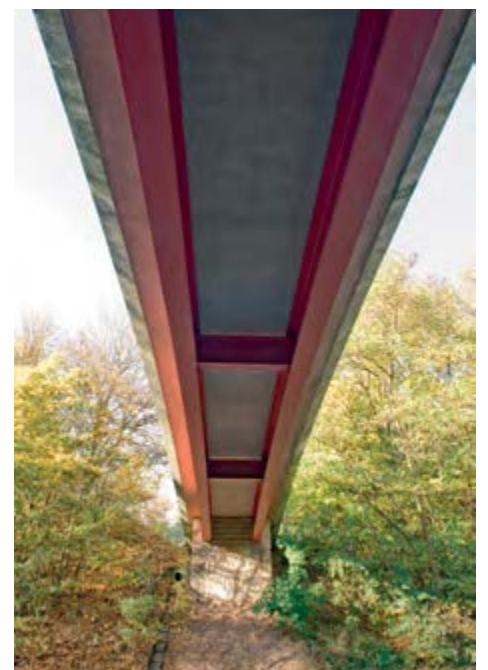
Bottom view on the twin-girder, composite footbridge at Wasserbillig, Luxembourg
