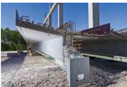
PreCoBeam used for the bridge at Vigaun, Austria.
