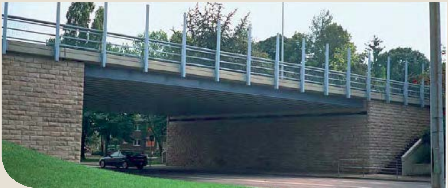
Filler beam deck bridge in Esch-sur-Alzette, Luxembourg – 19 m span; 0.65 m deck depth. For aesthetic reasons the edge beams are not encased in concrete on the outer side.
