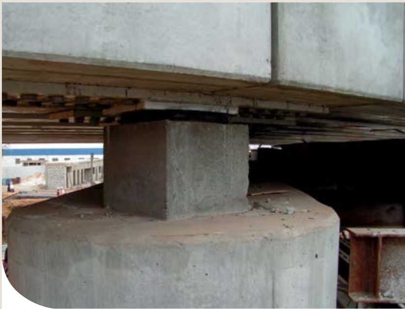
Pont de Cyrnos in Senegal - Detail of the support.
