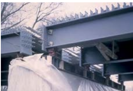
Bridge in Schwedt, Germany – Concrete connection of main girders.
