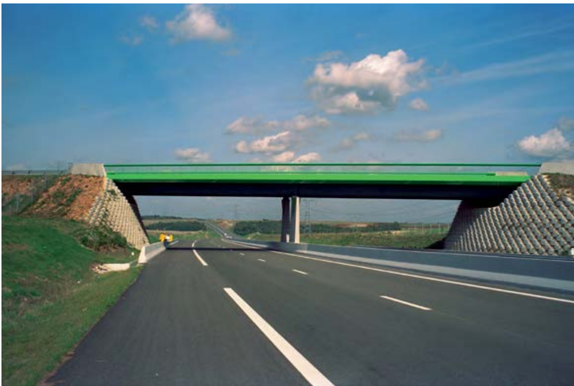
Road bridge over the A16 motorway, France - Composite deck with two main girders in high strength steel S460M.
