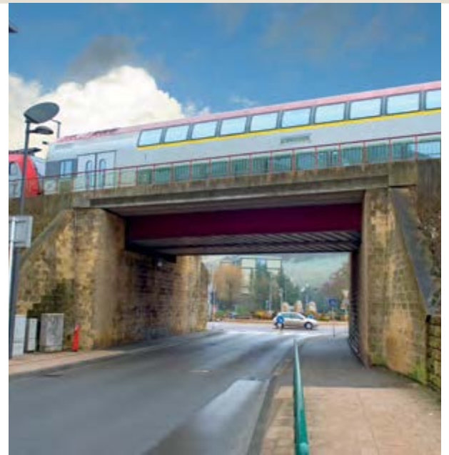
Reconstruction of the railway bridge over Emile Mark street in Differdange, Luxembourg – Because of the very restricted construction depth, two single track half-through type bridges were implemented.
