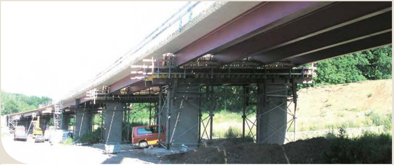
The Horlofftalbridge in Hungen (Germany) with eight spans constructed in 2006. For five spans partially prefabricated concrete beams with heavy rolled beams in S460 have been used.
