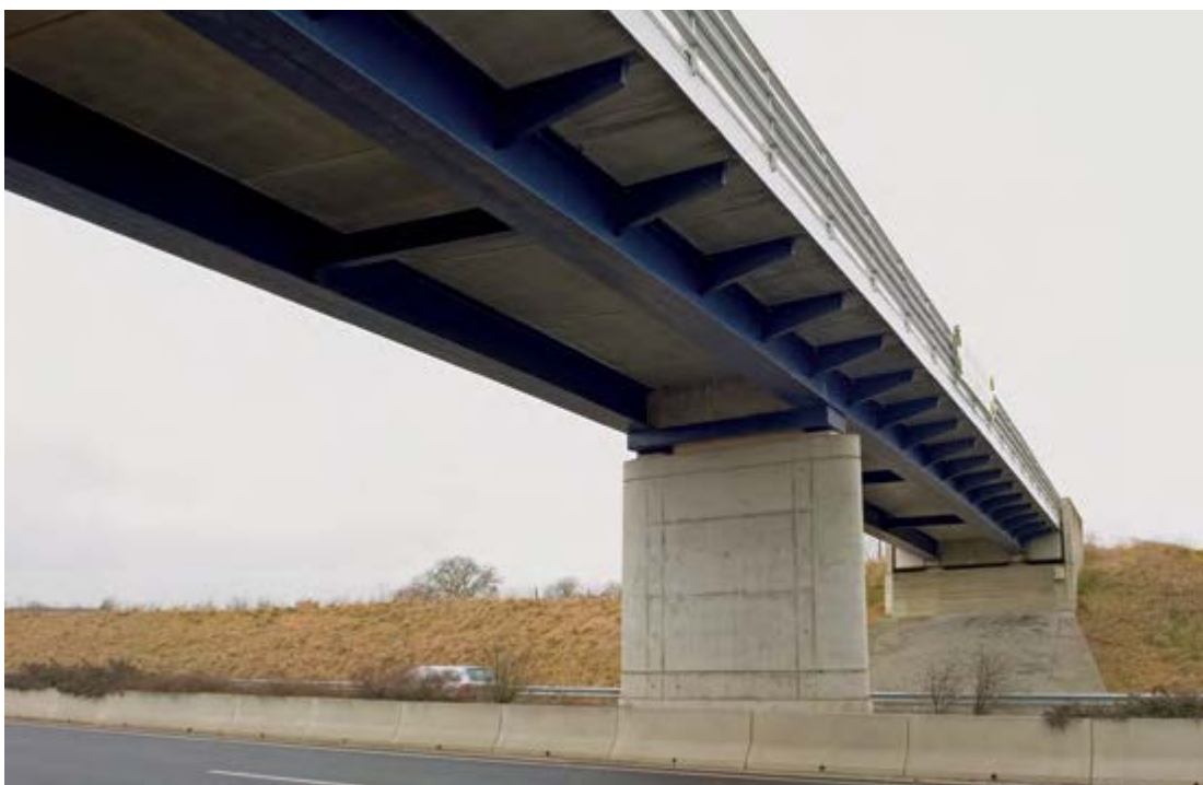
Bridge link to La Sarre, Luxembourg - The large cantilevers have been designed to support the prefabricated concrete elements during construction without any scaffolding, the box sections have been designed to resist the resulting torsional moment.
