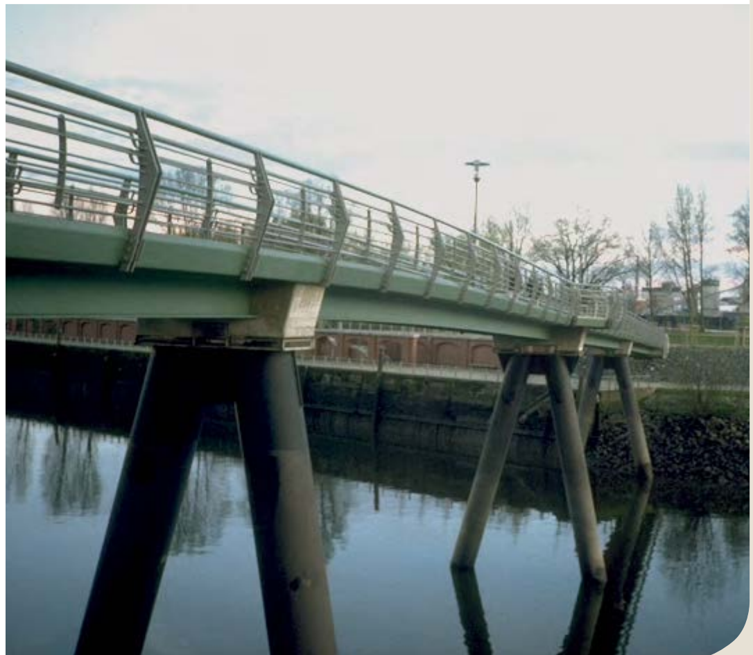
Footbridge over the Haken in Hamburg, Germany – Slender bridge with 4 spans of 25 m.
