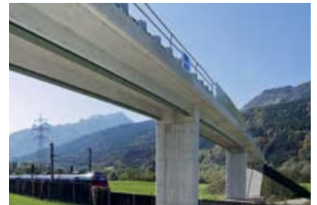
The Vigaun bridge made of PreCoBeams with three spans of 26.15 m and a slenderness ratio of 1/23.
