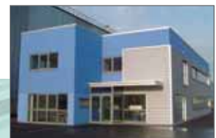
Eurostructures-Büro 49° 32' 16.6" N 5° 54' 39.0" E
