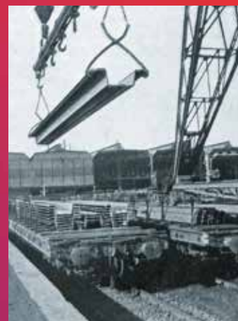
Belval steel works, Luxembourg, 1930s
