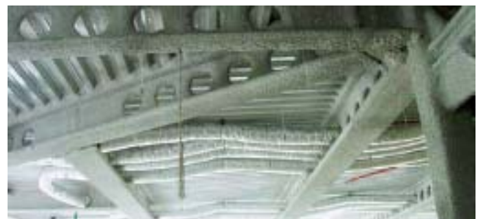
Figure 9.2: Protection by spraying on ACB® beam
