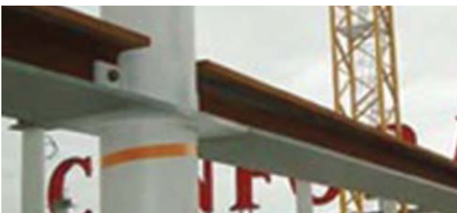
Figure 6.6: Slim-Floor for parking in IFB (Nantes, France)
