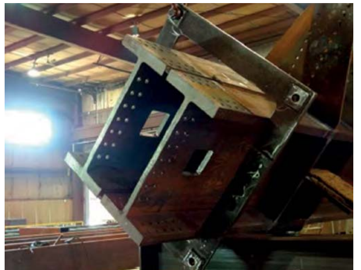
Figure 4.6: Two heavy sections welded together
