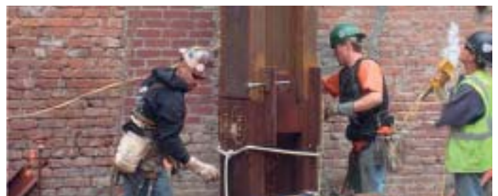
Figure 7.2: Column joint before welding
