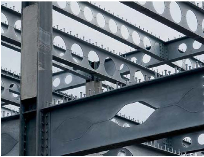
Angelina® beam with filled openings at support
