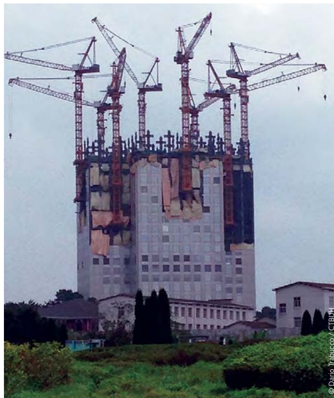
Figure 2.2: Broad J57 Tower, 19 days for 57 storeys, Changsha, China
