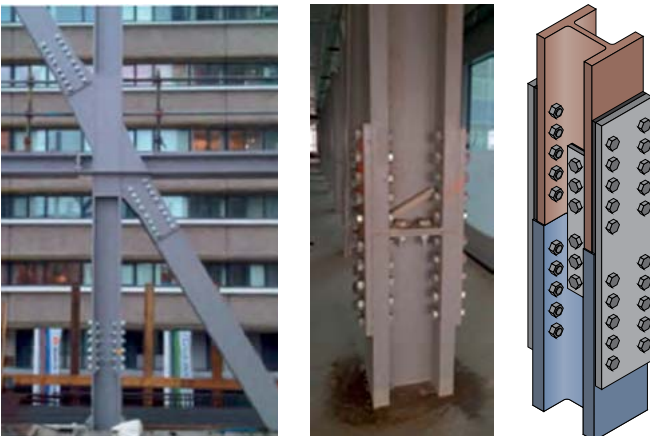
Figure 7.1: Bolted connection of two HD/UC/W columns
